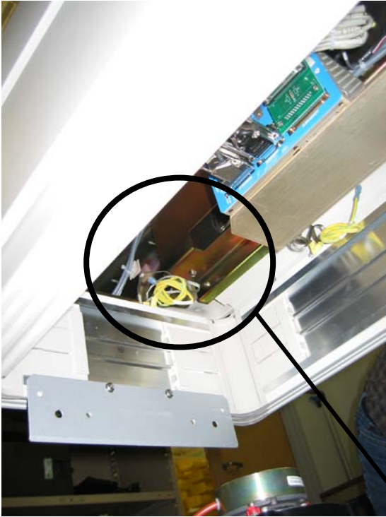
Figure 2: Underneath Rear of Sub-frame
