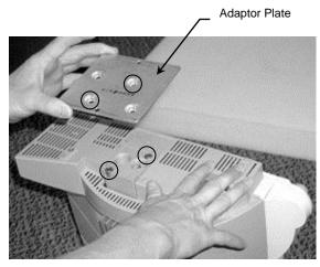
2. Secure the Adaptor Plate to the device by using the supplied M6 40mm FHMS (2).
